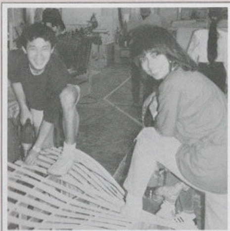
SMArchS students Kevin Low and Radziah Mohamad build form for catalonian vault.
