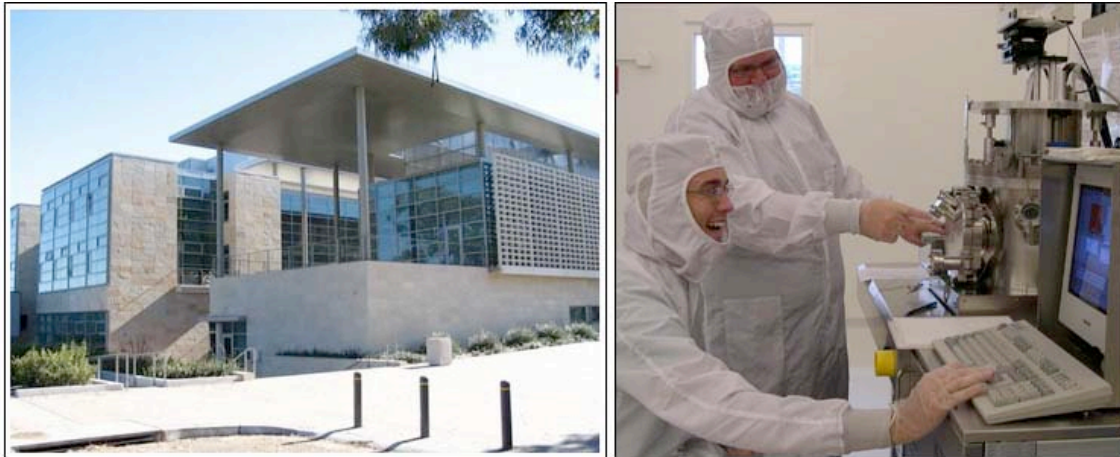
Figure 13.9. (Left) The new Engineering Sciences Laboratory which is home to the Nanofabrication Facilities (right) at UC Santa Barbara.
