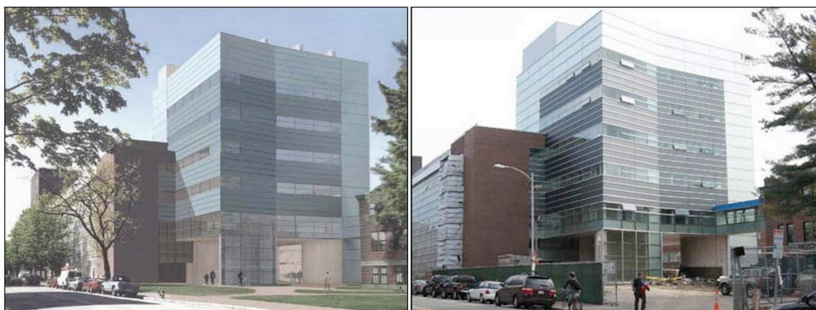
Figure 13.1. Computer aided design of the new Laboratory for Integrated Science and Engineering (LISE) building ( left ) and the completed building at Harvard University ( right ).
